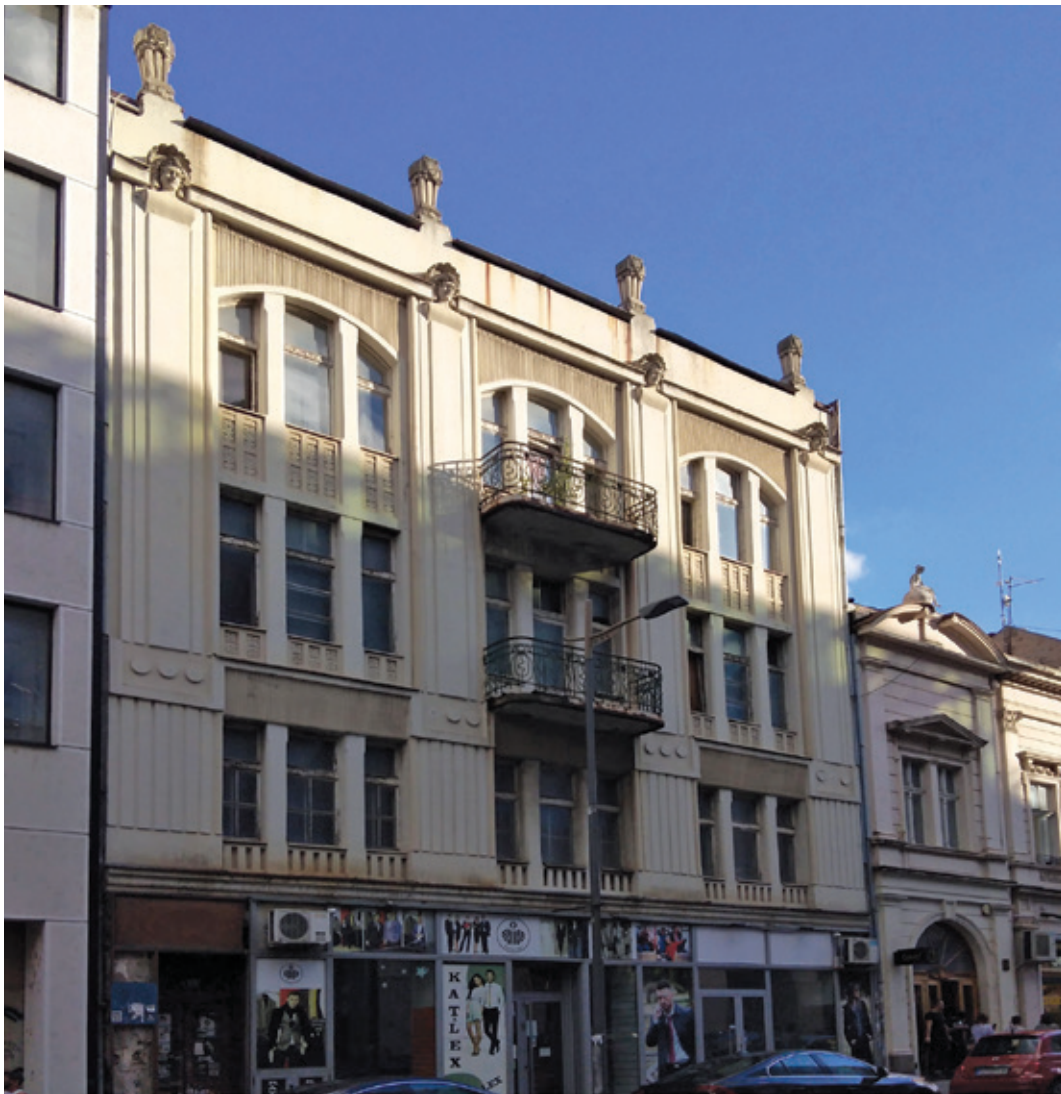
Fig. 4. Building for Josif Alkalaj (1920), exterior, 26 Kralja Petra Street (photo: Verica Pavićević)
