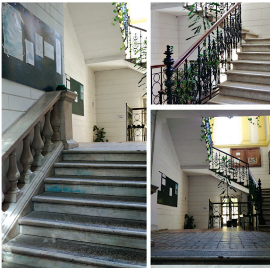
Fig. 1. Popović brothers' house entrance interior (1900), corner of Simina and Dobračina streets (photo: Verica Pavićević)
